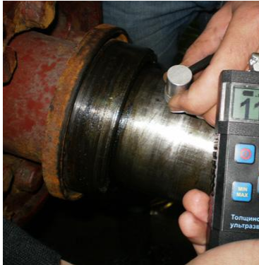
Measuring the thickness of the motor shaft
