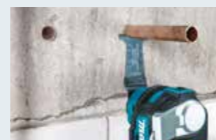
Copper pipe flush cutting
