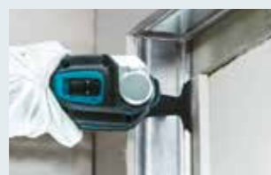
Door opening work
