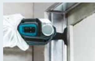
Door opening work
