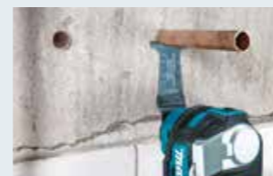
Copper pipe flush cutting
